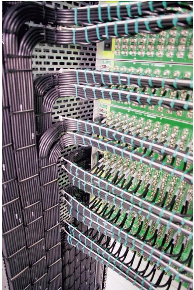
neat and bend the coaxial cable to match power and data cables on the tray must be avoided. Remember, **bending coax more than the minimum bending radius affects the impedance of the cable and causes a video signal quality loss**.
